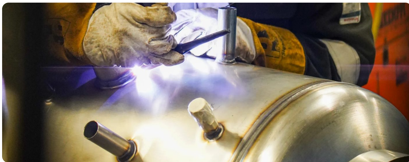
Welder joining a boss to a stainless steel vessel
